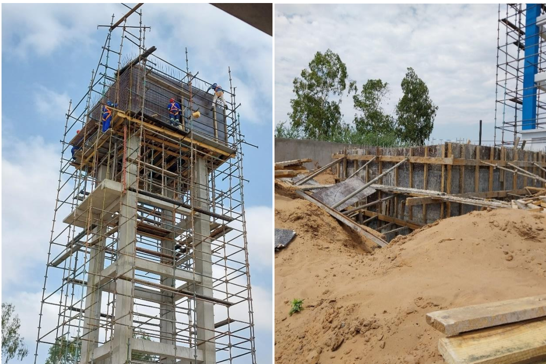
Figure 5. Water tower box and manager house slab formwork
