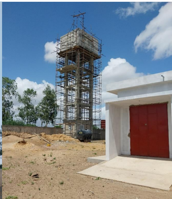
Figure 12. Unformed water tower box
