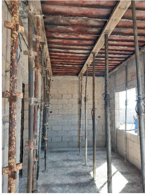
Figure 6. Bottom view of the assembled slab formwork
