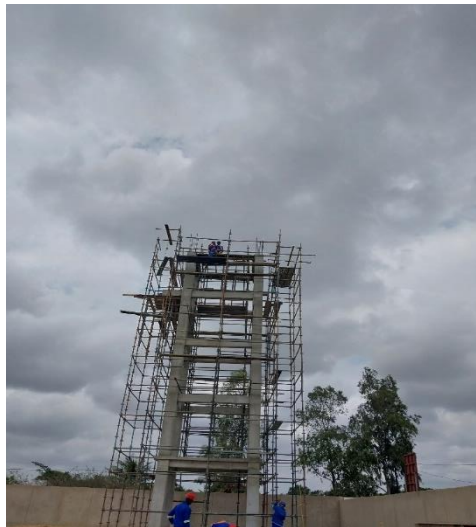
Figure 14. Concreting carried out by the bucket for discharging concrete
