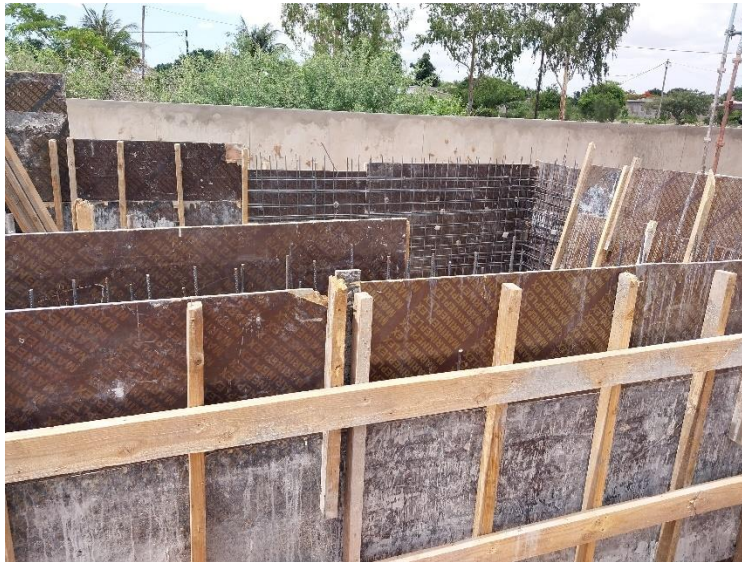
Figure 10. Frame and positioning of the mesh of the semi-buried deposit
