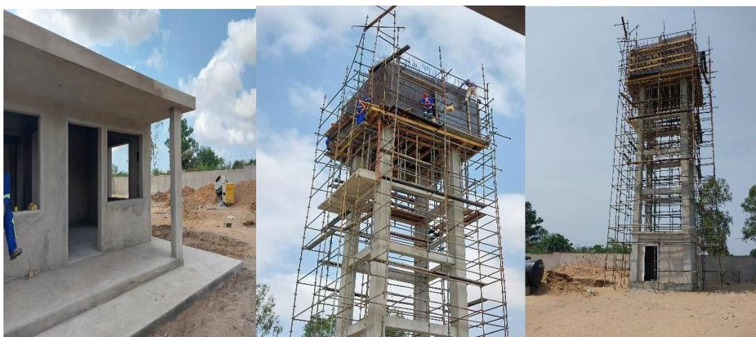
Figure 4. Construction of the case under study
