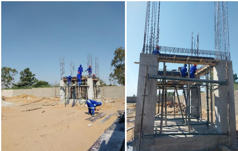
Figure 15. Water tower beam frame and formwork
