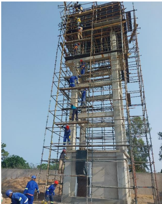
Figure 11. Concreting of the water tower box with the aid of buckets
