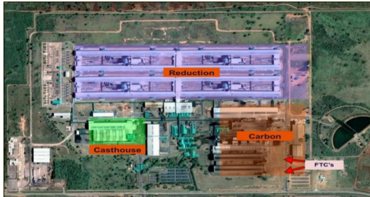
Figure10: Mozal Reduction Department overview (adapted from Mozal General Safety Induction Manual, 2019).
